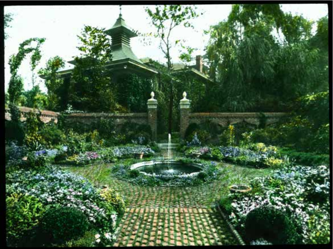
Slide 054—Mrs. Roy A. Hunt, featuring her garden at Elmhurst with her lecture text: The floor of the garden is almost two feet lower than the perennial border around the walls, and has a pool, copied from one of the Italian villa pools. The planting in the four beds is kept quite low. The color scheme is usually blue, lavender and soft pink. This slide shows the view from the little arbor toward the entrance gate.
